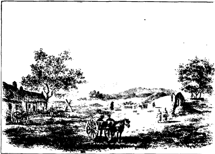
Fig. 15. Millburn Bridge near Moffat.
