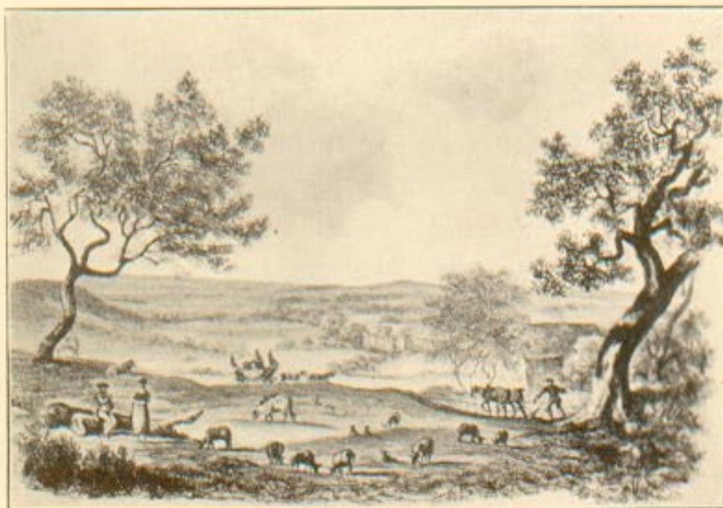
Fig. 12. New Road between Fiddler Bridge and Cartland Bridge.
