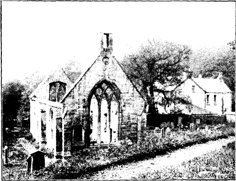
Fig. 17. Temple Old Church, from the South-east.
