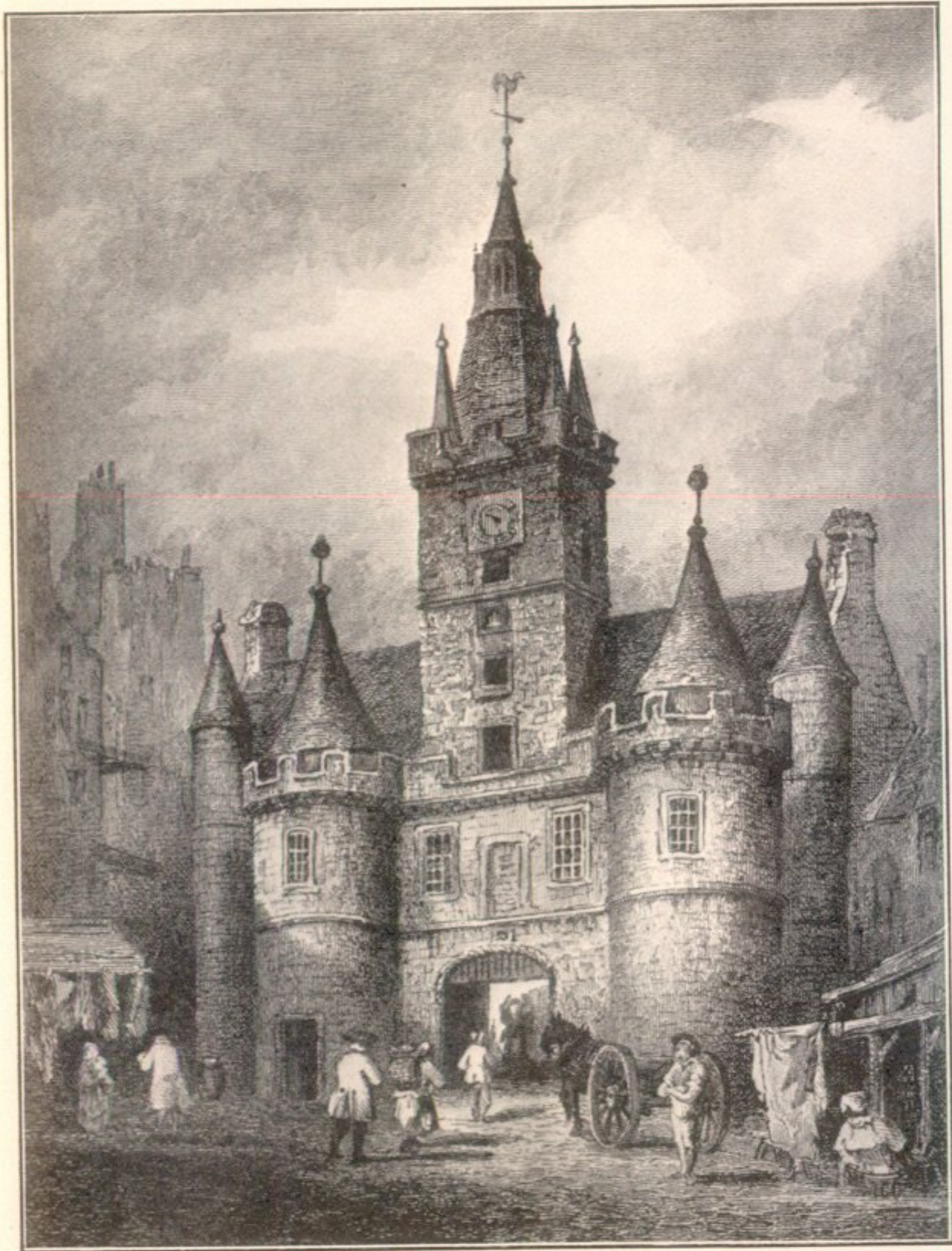
Fig. 2. The Netherbow Port from the east.
