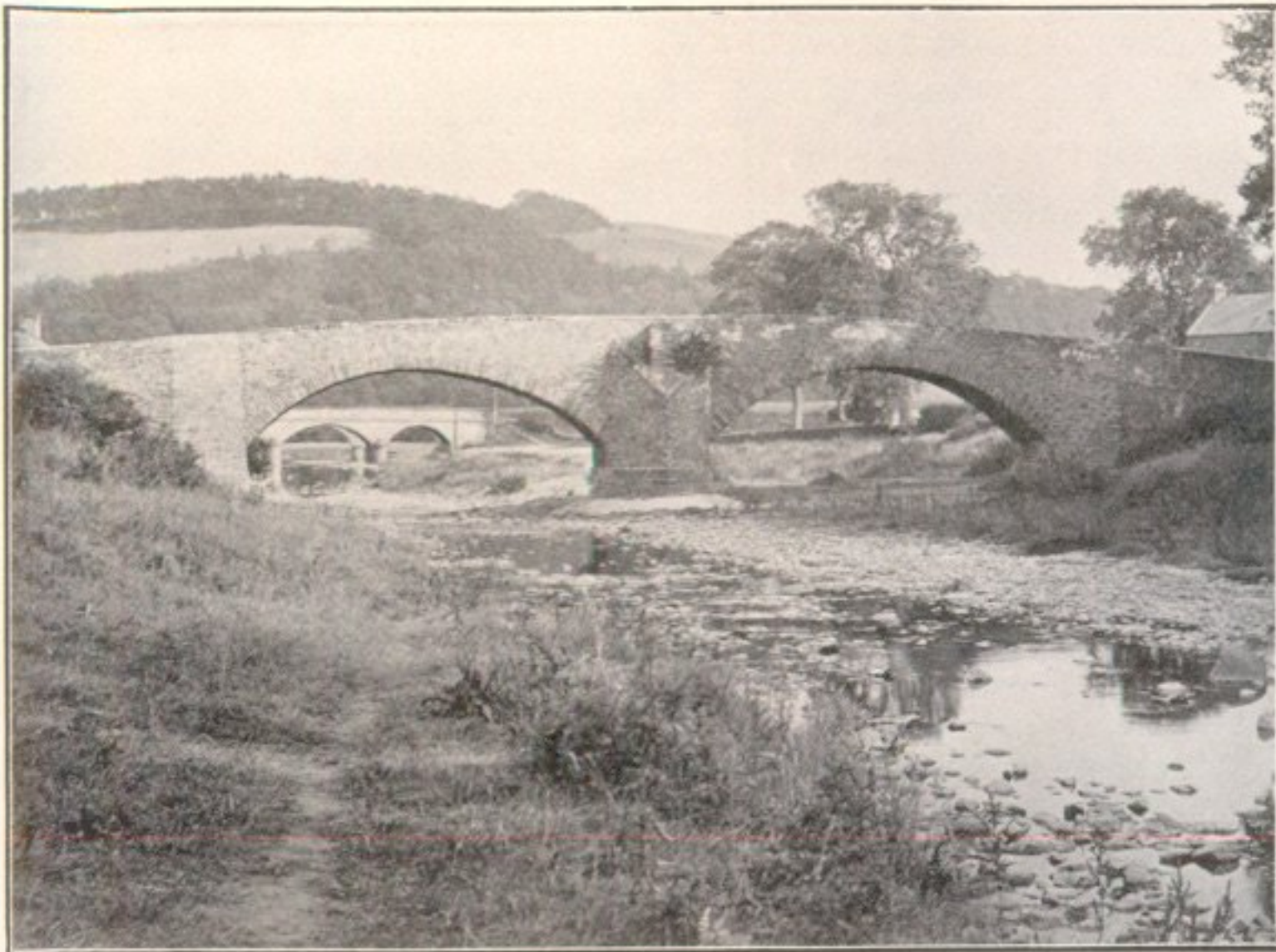
Fig. 12. Shire Bridge Period. Earlston Old Bridge; 1755. Roadway, 10 feet.
