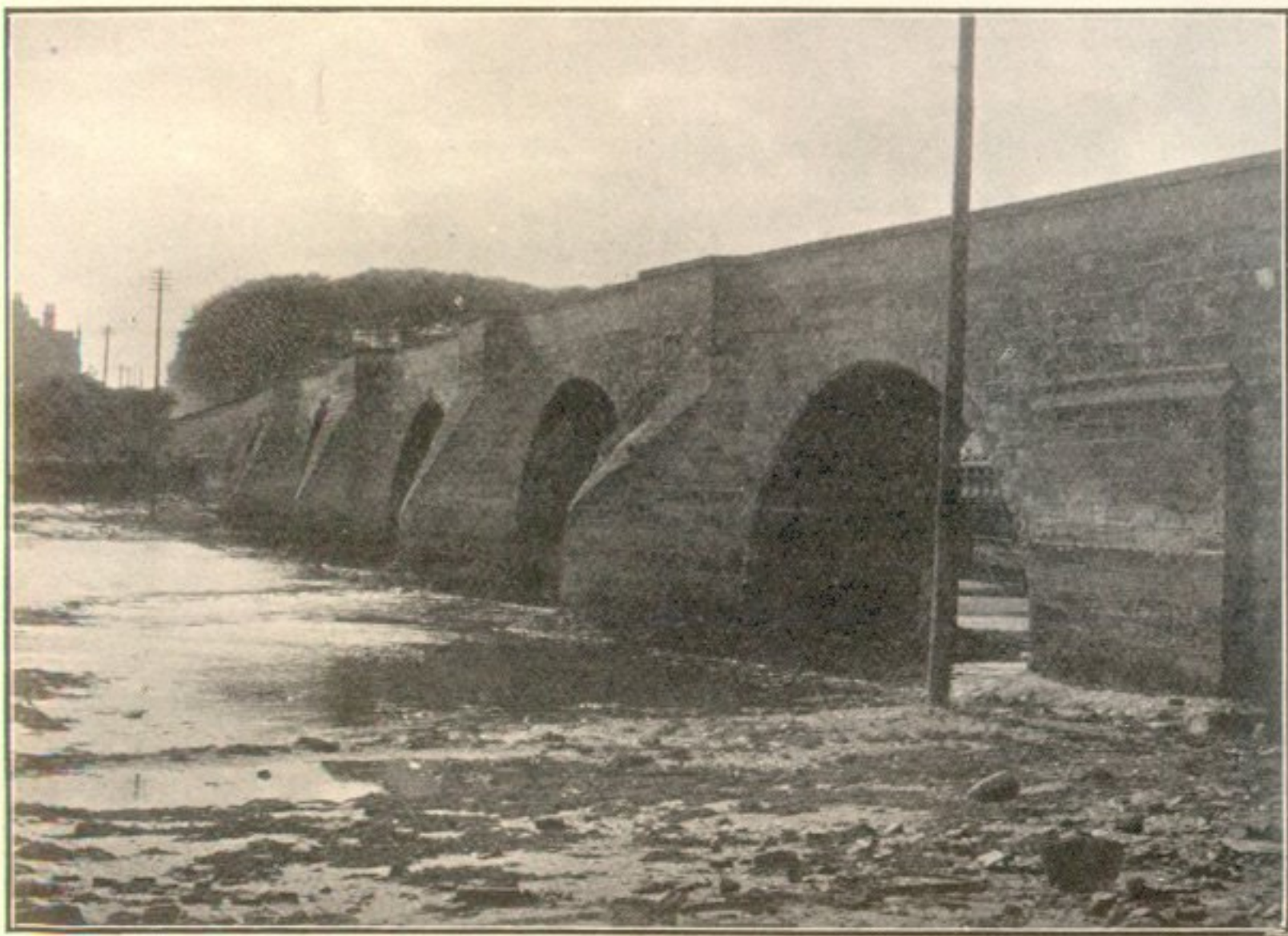
Fig. 8. Guard Bridge, St Andrews (1420–1530), showing the higher cut-water of the first Pier, and the low cut-waters of the older Piers. Roadway, 11 feet 6 inches.
