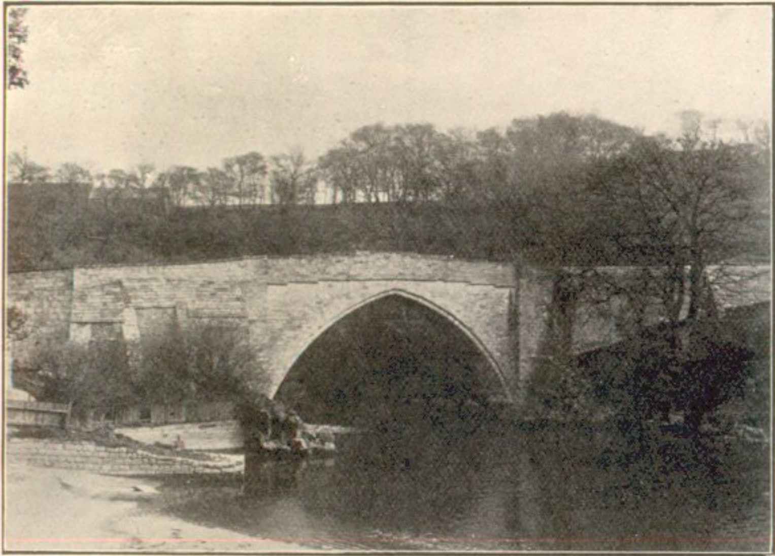
Fig. 7. The Brig of Balgownie (Aberdeen), reputed cir. 1320, but partly rebuilt 1597. Roadway, 11 feet.
