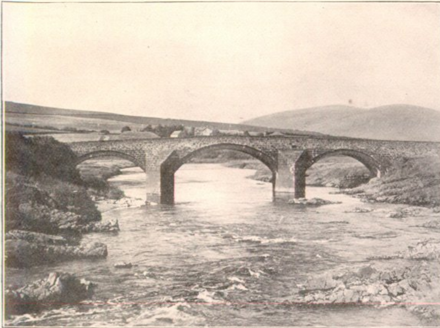
Fig. 14. Early Turnpike Period. Clydesbridge, near Abington; 1769. Roadway, 11 feet 9 inches; replacing an older Bridge.
