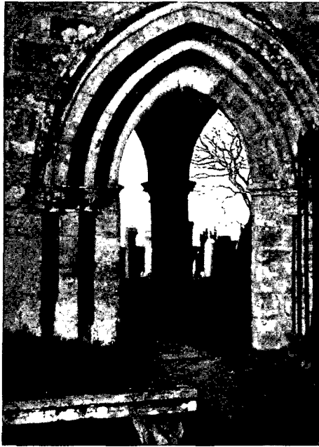
Fig. 2. Doorway in South Wall. (From a photograph by Rev. W. W. Dawson.)
