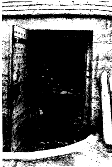
Fig. 28. Interior of Vault in Udney Churchyard, showing Inner Iron Door (partly raised) and Circular Revolving Platform.
