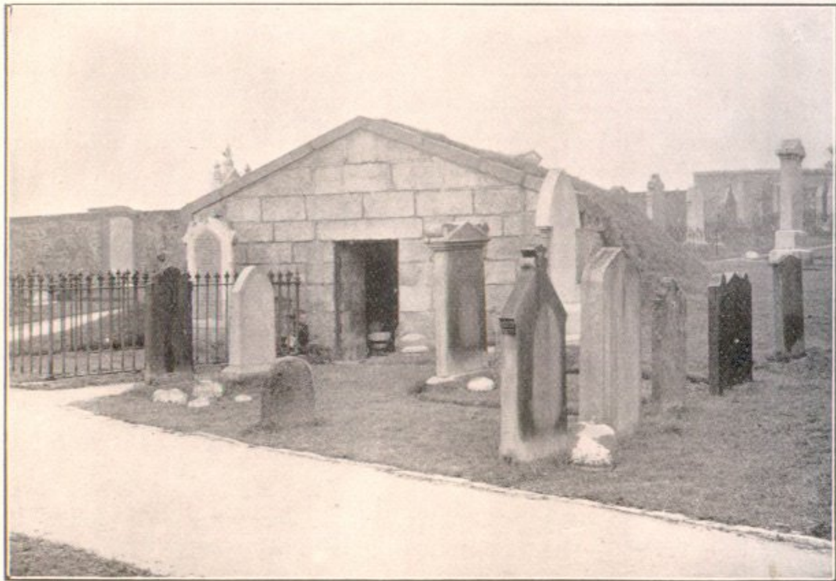
Fig. 19. Vault in Kemnay Churchyard.
