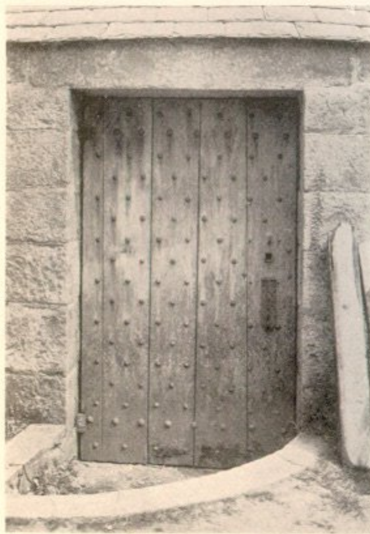
Fig 27. Outer Oaken Door of Vault in Udny Churchyard.
