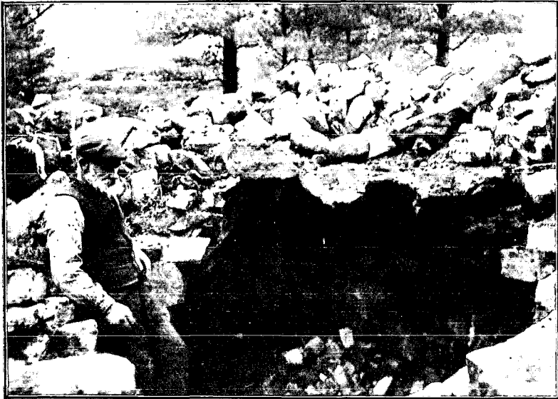
Fig. 3. View of the Chamber with part of the roof removed.
