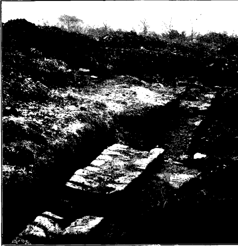
Fig. 13. Partition Wall in Praetorium, showing subsidence on line of Agricola Ditch.
