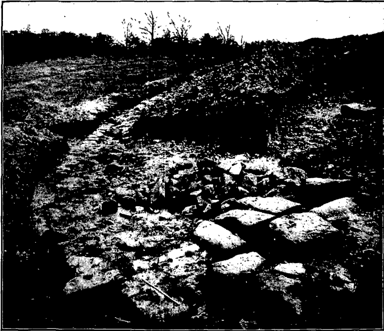
Fig. 6. Foundation of Rampart, N.E. corner, showing Conduit.
