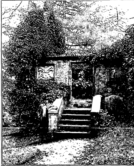
Fig. 2. Stair and Entrance to Transept.
