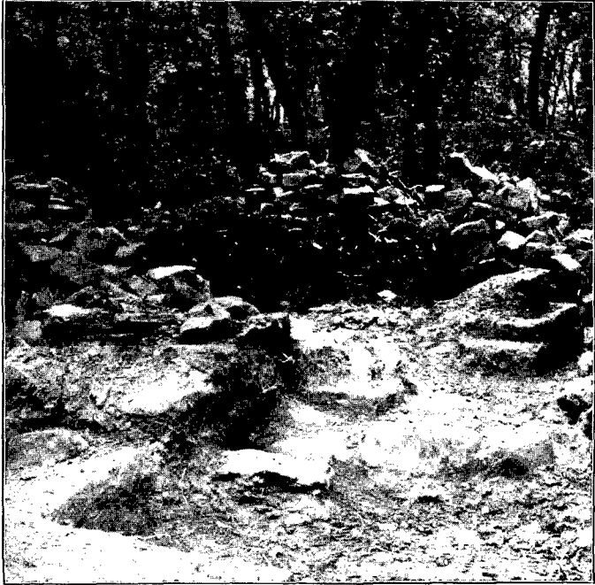
Fig. 19. Exit for water between Buildings No. 1 and No. 2.
