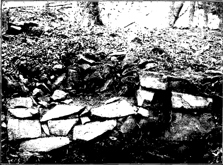
Fig. 10. Remains of the outer face and rubble core of the Wall, Duntroon.
