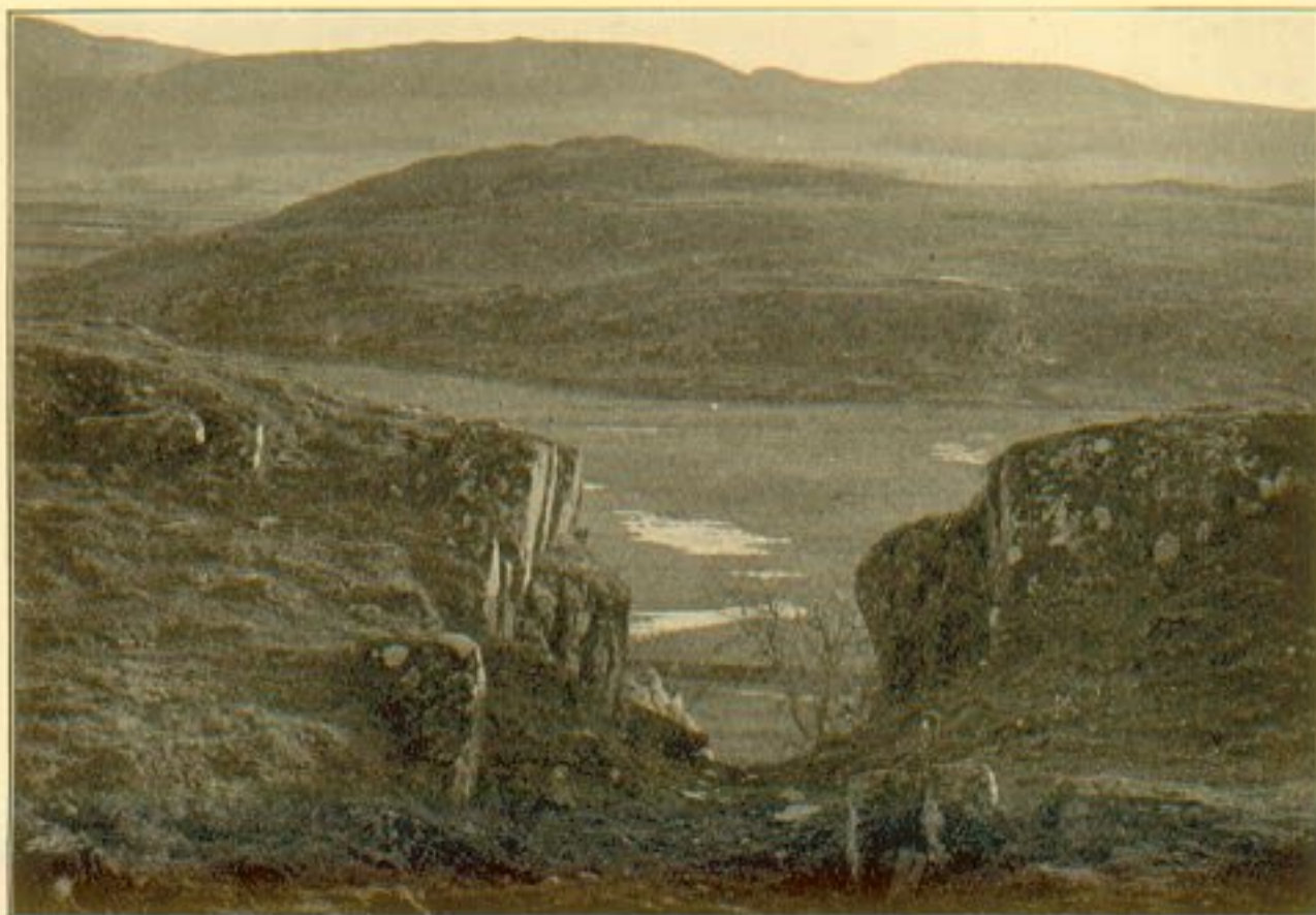
Fig. 26. Entrance to the Lower Fort, Dunadd, looking out.
