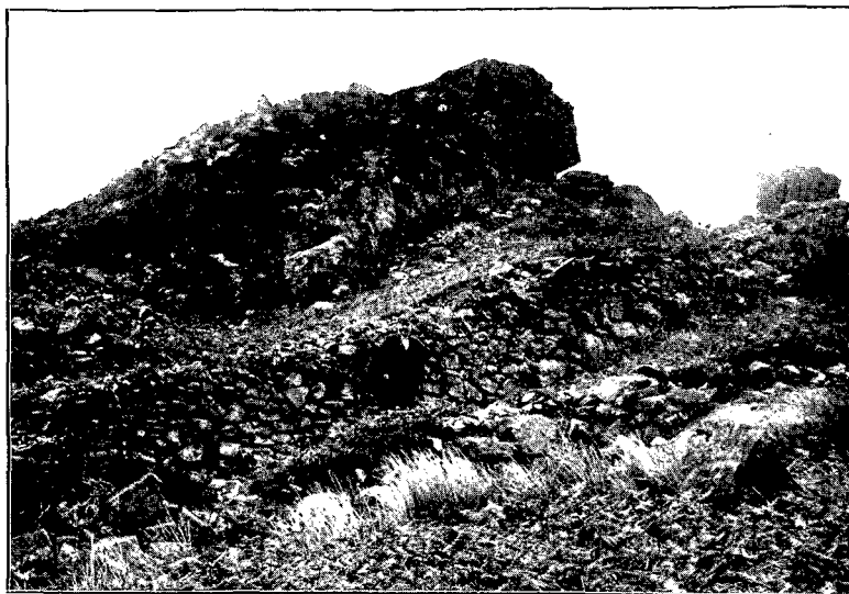
Fig. 5.—Rhu Varkie, showing masonry of the middle and exterior walls.
