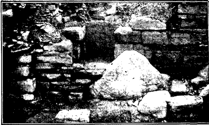
Fig. 9. Keiss Broch. Closed entrance on east side, with part of slab door in situ , and triangular stone at base of outside wall.
