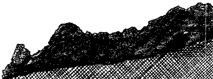
Fig. 5. Elevation of Vitrified Wall of Dunagoil.
