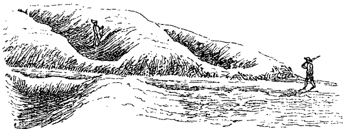
Fig. 71. Entrance to Harehope Fort.
