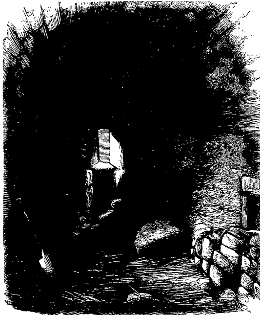
Interior of the building, showing splayed window in eastern gable, recess in interior of south wall, vaulted-roof, &c.
