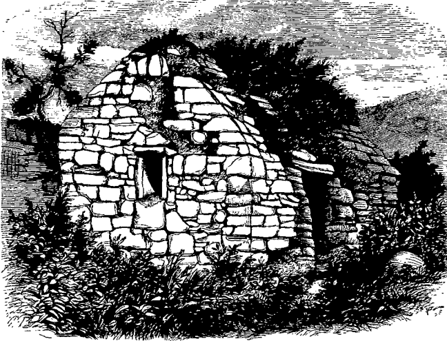
Eastern gable and north side of the building.
