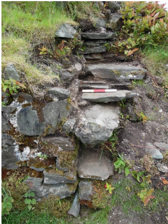
ILLUS S8 & S9 Straight Joint 2 from the north-east (left) and from above (right). The cross-wall clearly abuts the internal face of the inner bailey NW curtain wall, and this has aided its survival. Scales 300/100mm.
