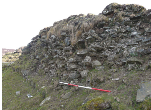
ILLUS 9 Part of the cross-wall from the north, highlighting a large volume of upstanding core rubble and some fragmentary areas of wall facing at current ground level. (© Mark Thacker)
