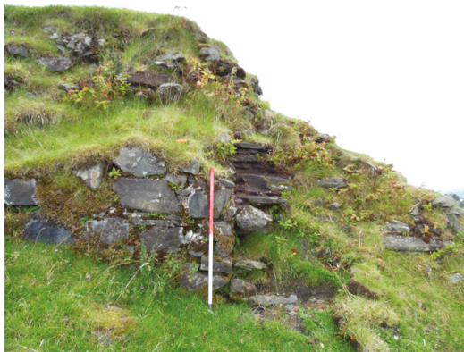
ILLUS 7 Straight Joint 2, from the north-east. Importantly, this straight joint aligns with the internal face of the inner bailey north-west curtain wall, here fossilised by the abutting cross-wall. This image also highlights the contrast in survival between the cross-wall (left) and curtain walls (right) in this part of the site. (© Mark Thacker)
