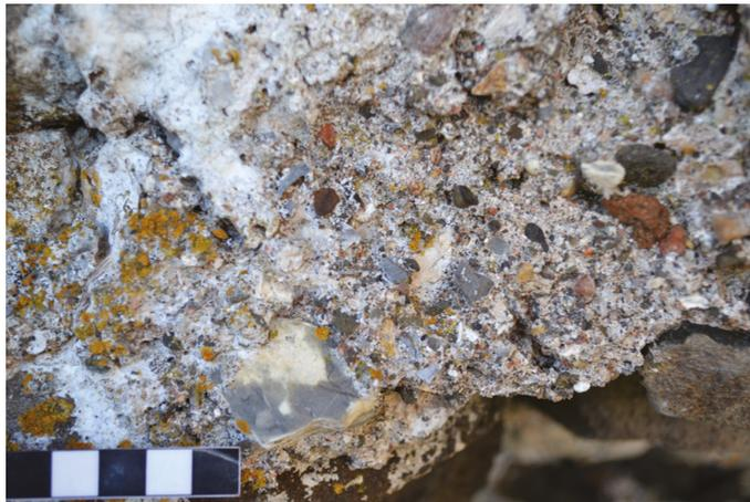
ILLUS 10 Mortar 1 in core of east wall of north-west block. Note the large sub-angular probable limestone kiln relict close to the scale strip. Scale 10mm
