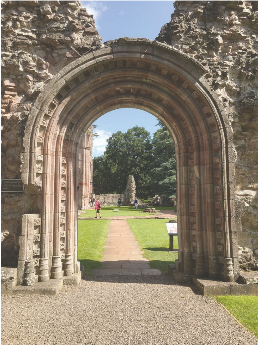
ILLUS 4 Dryburgh, west doorway. This view shows rough internal wall packing exposed by removal of the abbey's ashlars, a process halted by Buchan's acquisition of Dryburgh in 1786. The sculptured doorway itself – probably 15th century Romanesque revival rather than 12th century Romanesque – had been less desirable for re-use than the ready-made flat-faced ashlars. (© Aonghus MacKechnie)
