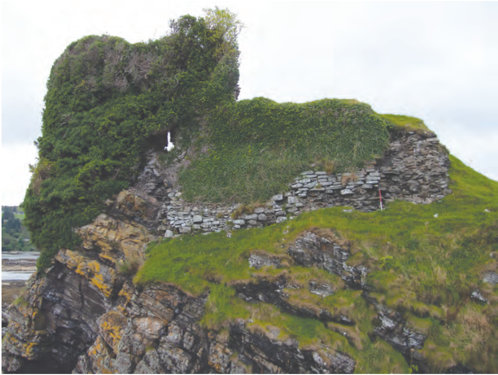
ILLUS 5 The south-east range from the south-east, 2014. Note the flat-laid faces and uncoursed character of exposed external masonry at low levels. (© Mark Thacker)
