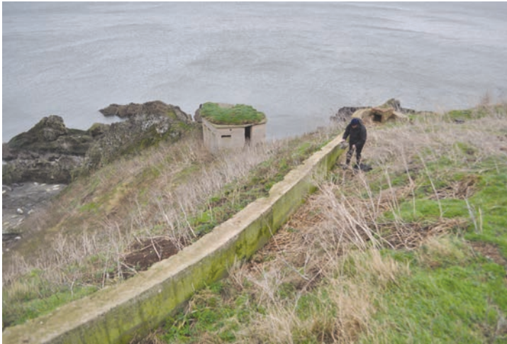
ILLUS 12 Concrete-walled firing position on Inchkeith, built before 1911. A First World War blockhouse (No. 8 using the 1918 numbering) is visible behind (Authors)
