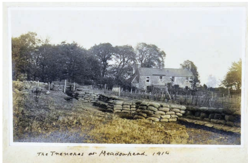
ILLUS 38 A photograph of the defences immediately south of Meadowhead farm, Liberton. The firing positions take the form of a trench fronted by a loopholed sandbag parapet. They are exactly as shown on the contemporary map (Major D Huie)
