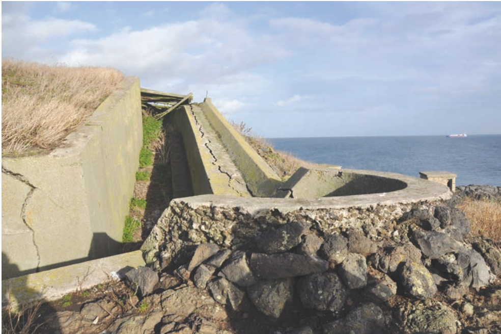
ILLUS 13 The concrete-lined, timber-roofed firing trench built across the south front of the South Fort on Inchkeith by the time of the 1911 map (Authors)
