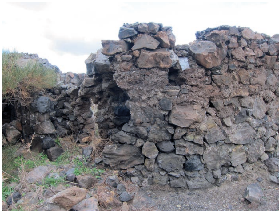
ILLUS 10a Upstanding remains of the wall of one of three upstanding calcarone furnaces, consisting of external and internal stone masonry wall in-filled with rubble. The interior wall is lined with plaster. © The Vulcano Project
