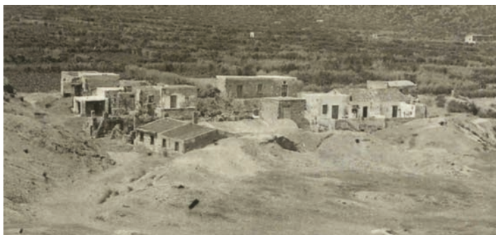
ILLUS 5b Detail of the state of preservation of the 'workshops' (some roofless, others abandoned but a few restored and referred to as 'farmhouses'). Photograph dated 1922, detail from photograph by L Sicardi, published in Giustolisi 1995, fig 48
