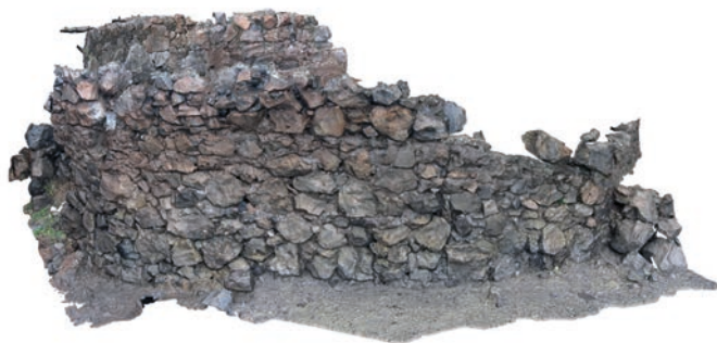
ILLUS 10b 3D photogrammetric model of part of the front wall giving great detail of the construction materials and ore waste embedded within. © The Vulcano Project
