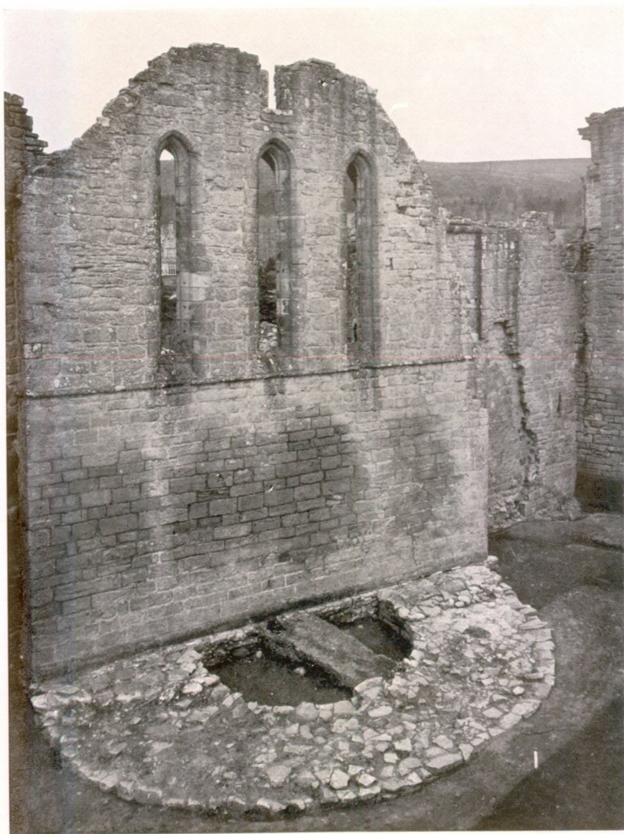
Chapel gable and abutting foundation
