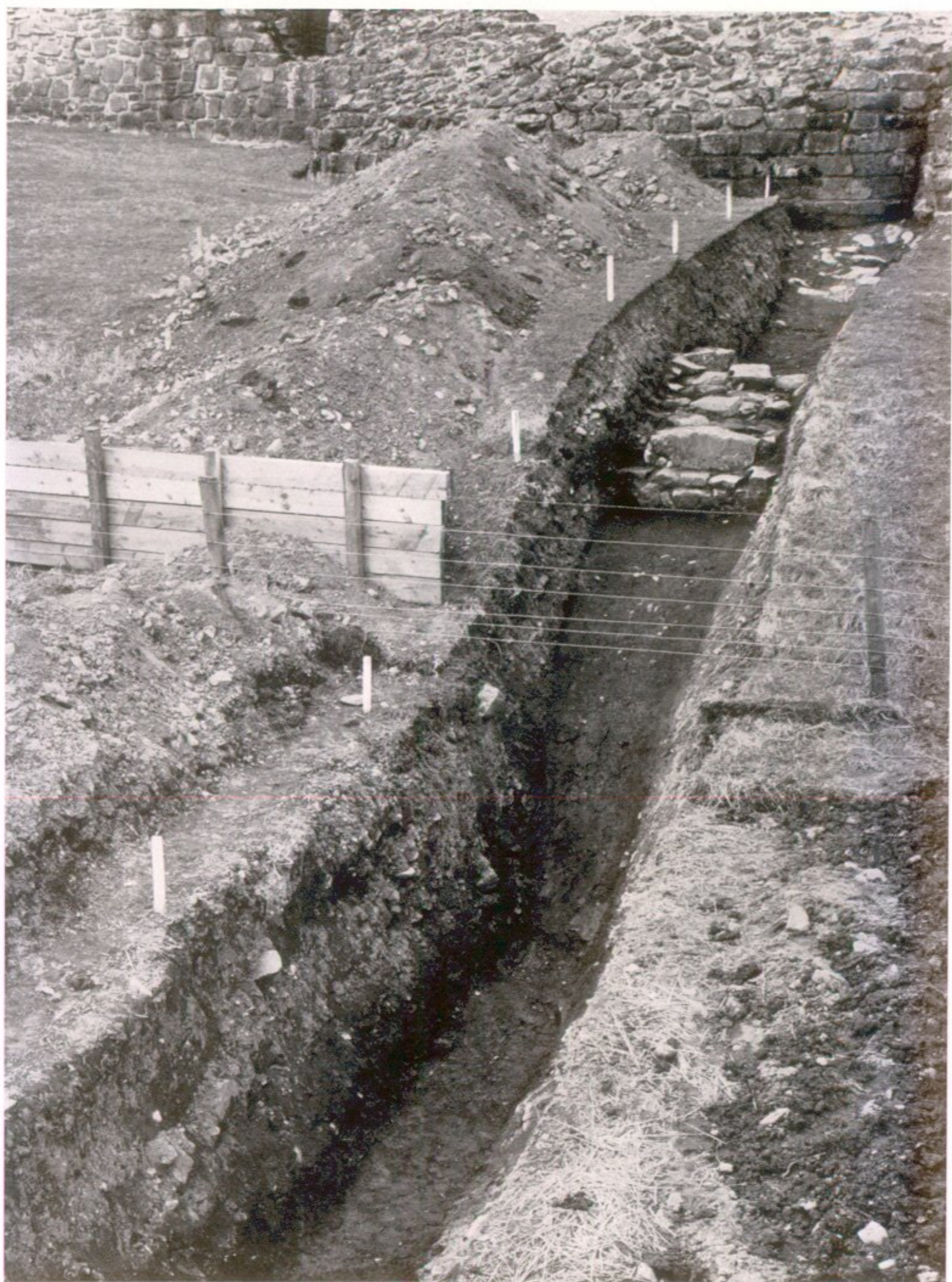
Ditch and outer wall S. of castle
