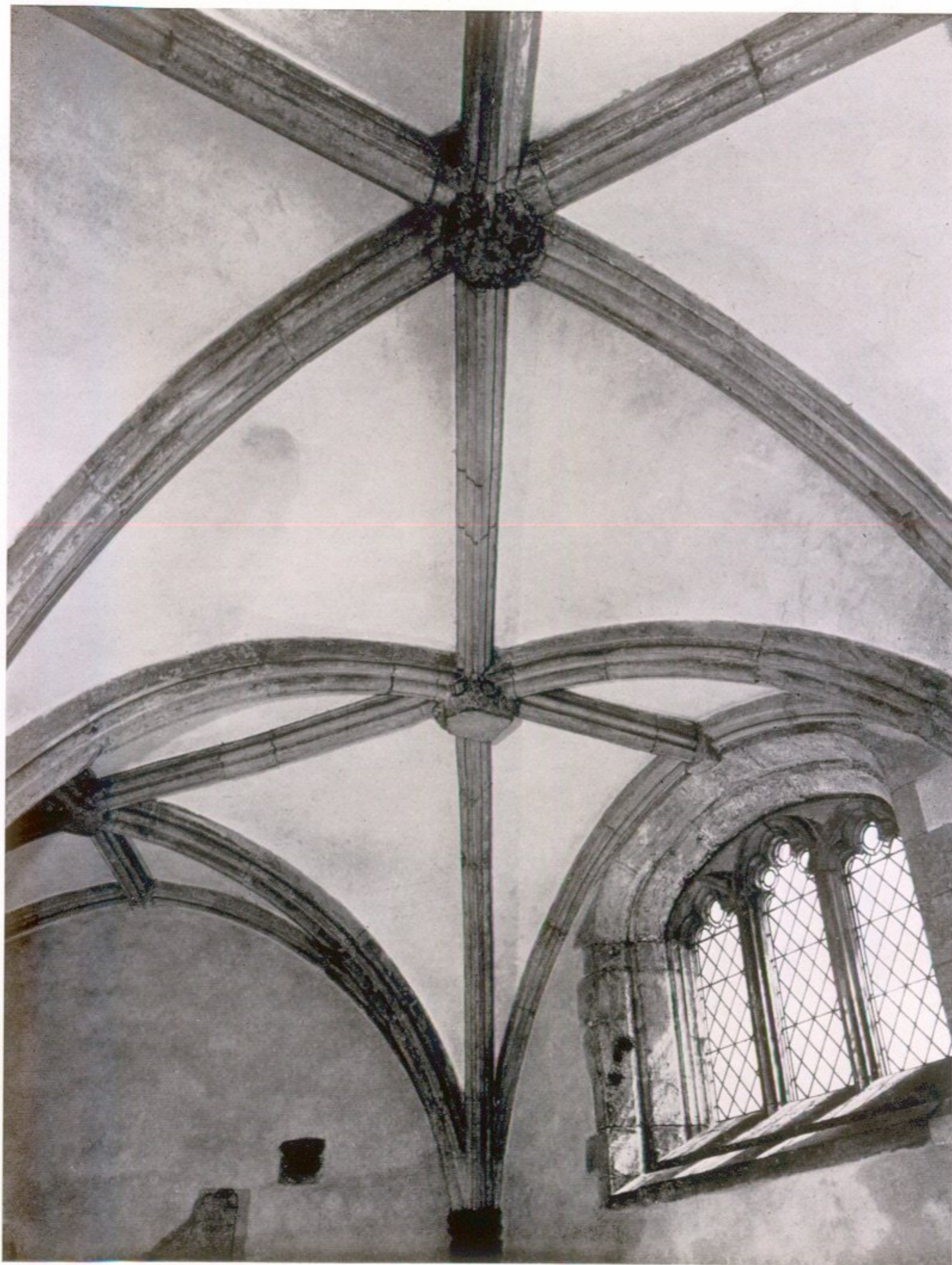
Lower Chamber: vault panels re-harled
