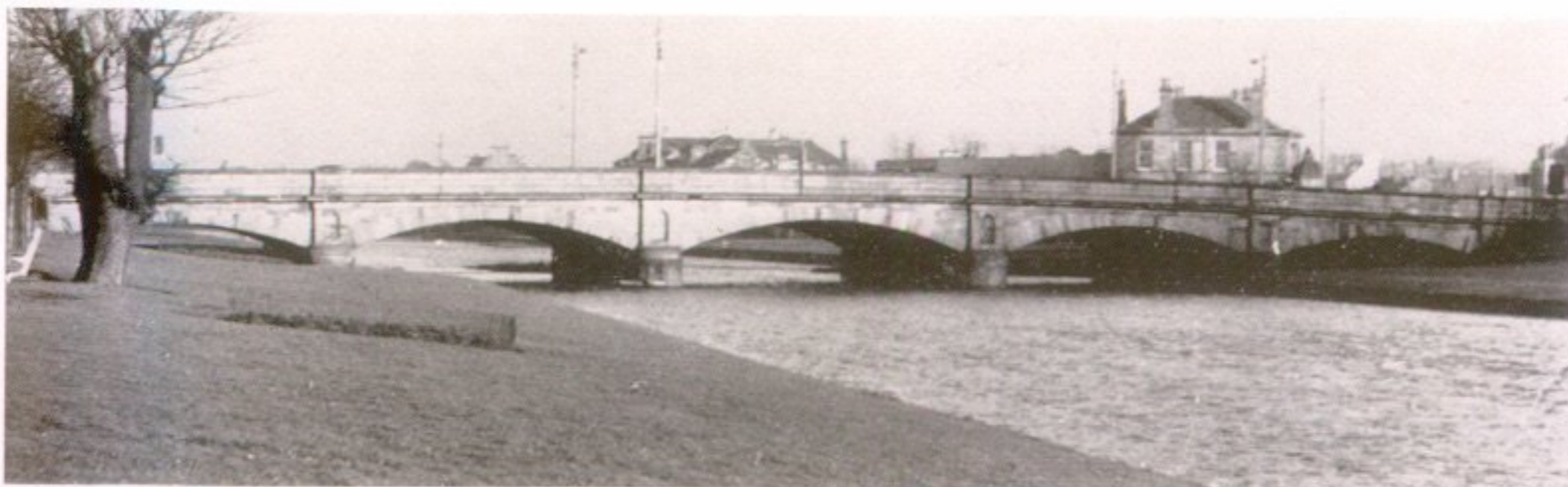
1. Musselburgh Bridge (1807), upstream side
