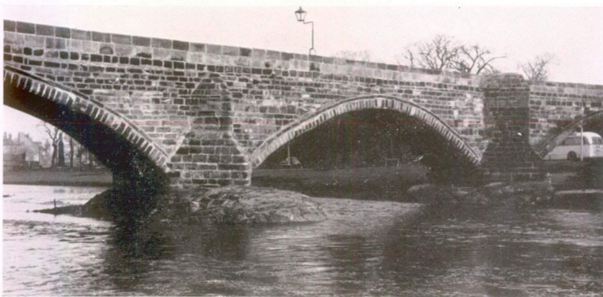
2. Musselburgh Old Bridge (mid-sixteenth century), upstream side
