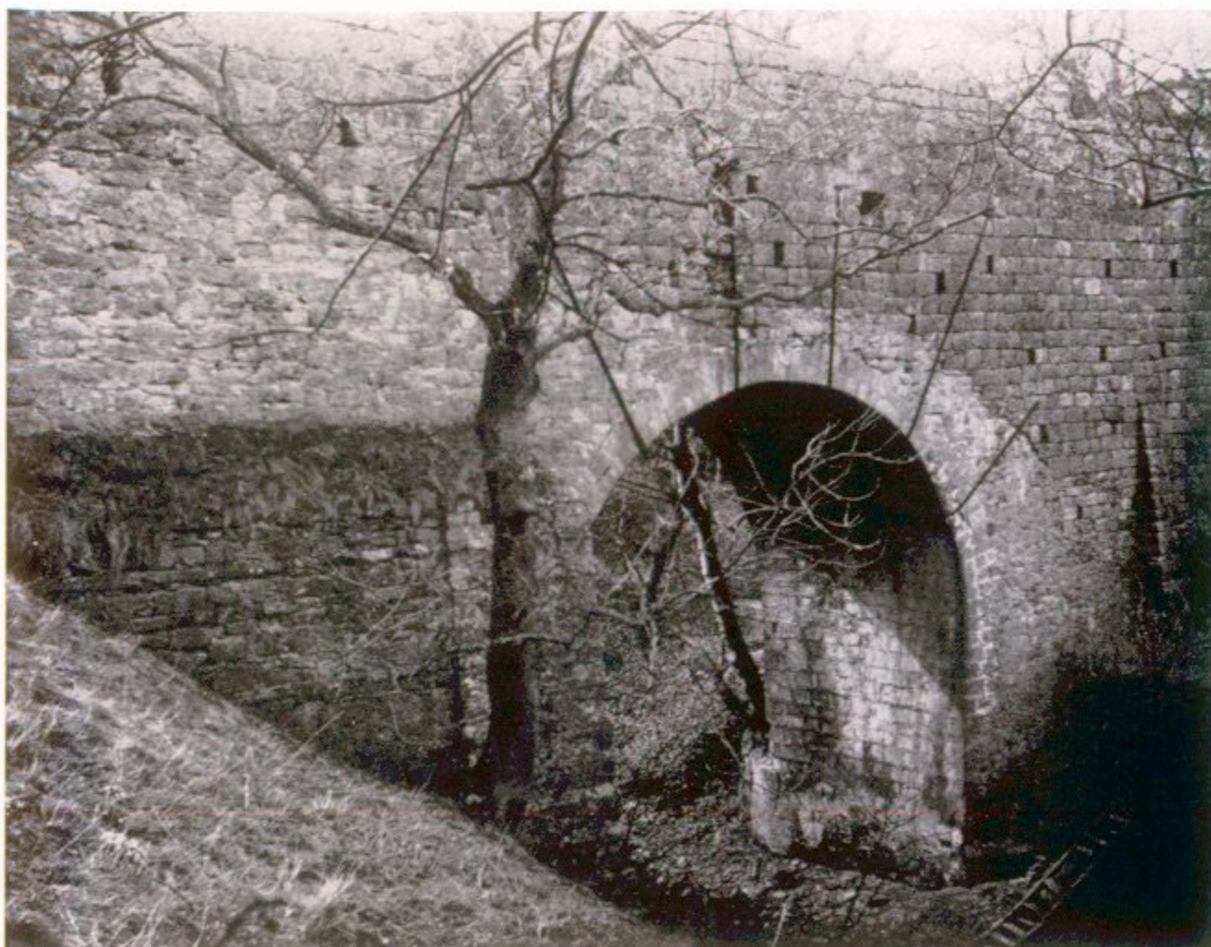
1. Dunglass Old Bridge (seventeenth century), downstream side
