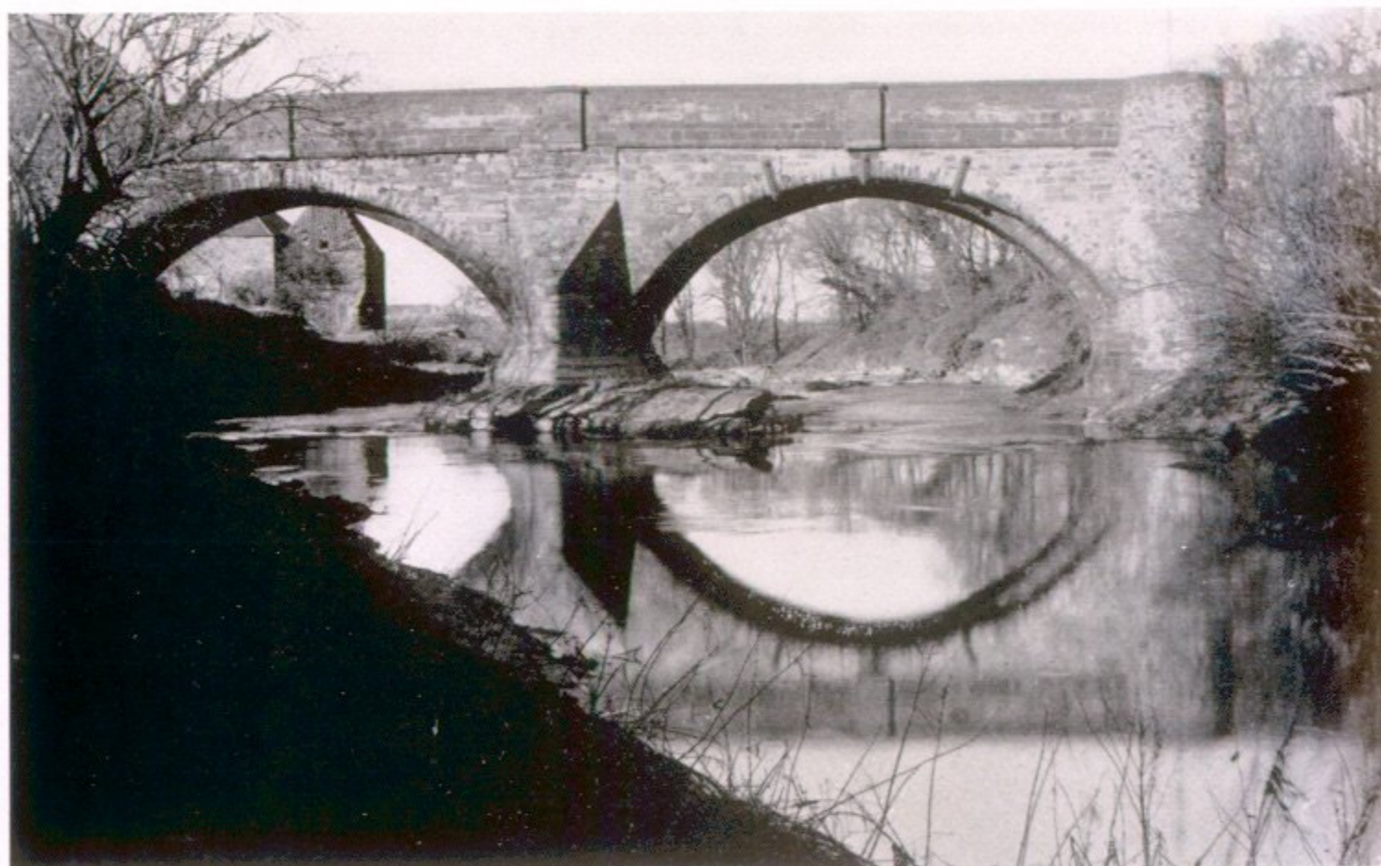
1. East Linton Bridge (mid-sixteenth century), upstream side
