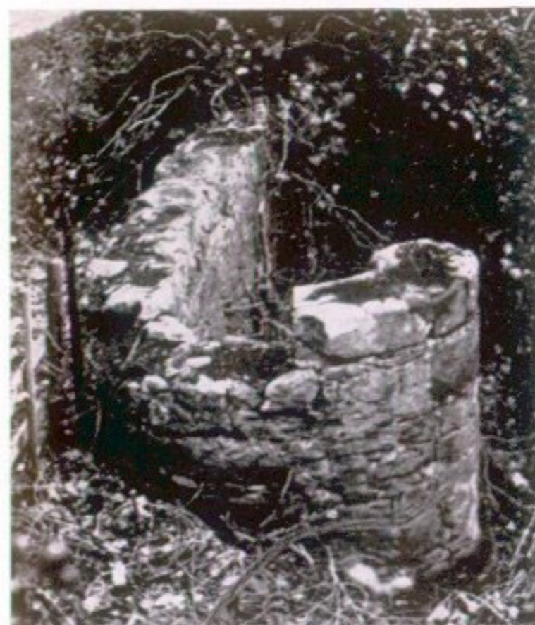
2. Dunglass Old Bridge; W. terminal of the upstream parapet
