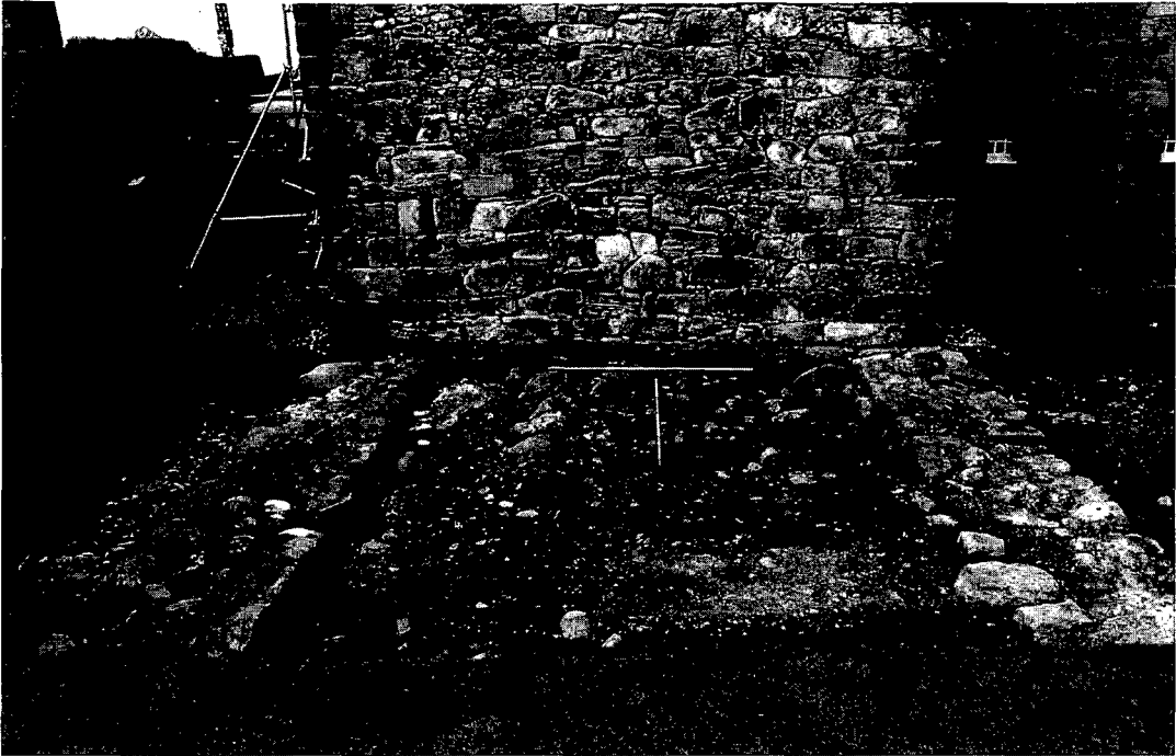
ILLUS 5 Trench A viewed from the south. Note the dumb-bell gunloop in the south wall of the gatchouse, sighted along the outside of the barmkin wall but blocked when wall F09 was built to its immediate west
