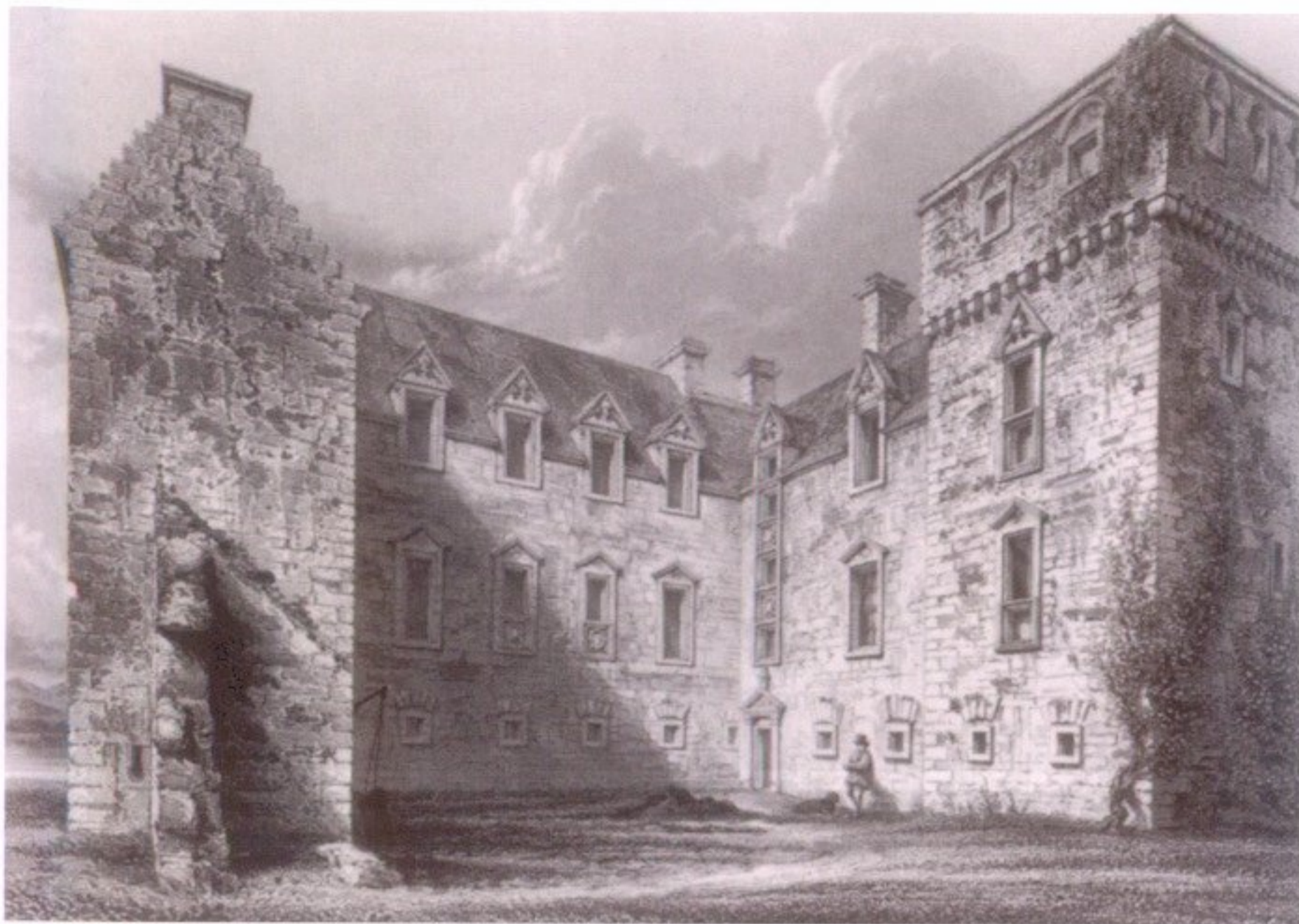
ILLUS 10 Drawing of Newark Castle in the mid 19th century, by Robert Billings (1852, pl 24), showing the remains of the barmkin wall against the south wall of the gatehouse; note the gunloop sighted along the outside face of the barmkin wall
