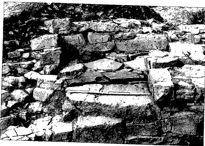
Illus 11 Broch entrance passage, looking east from the internal courtyard
