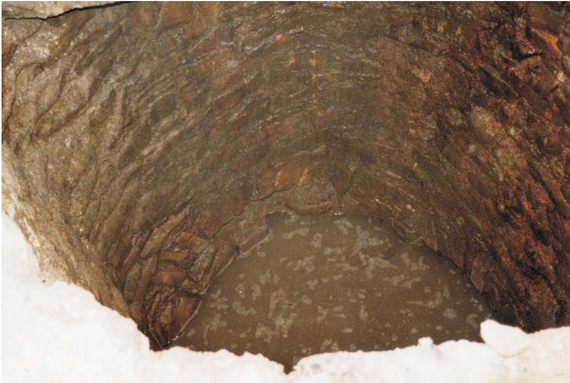
Illus 9 The well at the Black Bull, showing the two vaulted feeder drains
