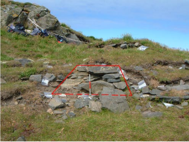
Illus 35 Erosion scar F on Dun Arnistean from the west. Scale 0.3m long.
