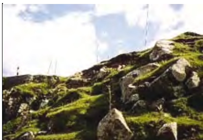
Illus 103: SFS 30, An Corran C: view of erosion face from below; NGR NG 4877 6840
