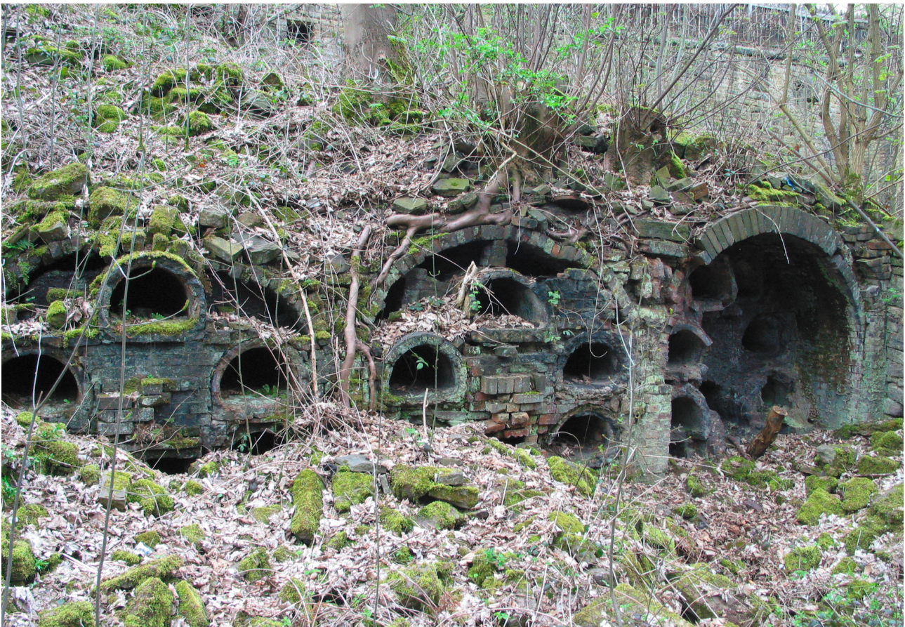
Illus 87 Ceramic retorts at the abandoned gasworks site at Shaw Lodge Mill, Halifax
