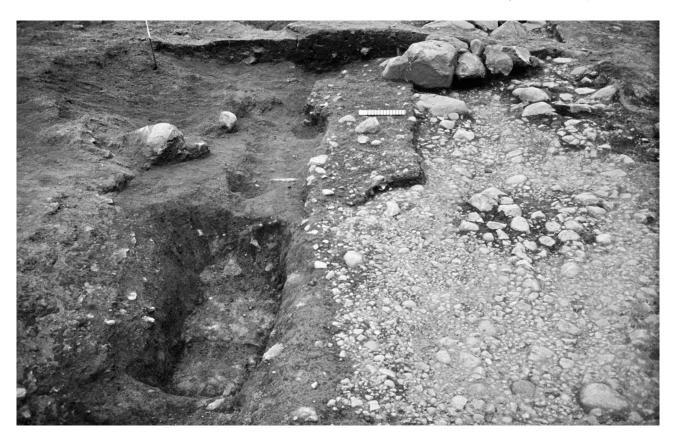
**Illus 4.4** Well-preserved section of metalling of primary road surface and associated drainage ditch (CCK) immediately to the west of intersection with link road to the fort, from south-west. Some large displaced kerbstones and a patch of later damaged metalling are apparent (top centre), with a probable pothole repair to the primary surface (centre right)
