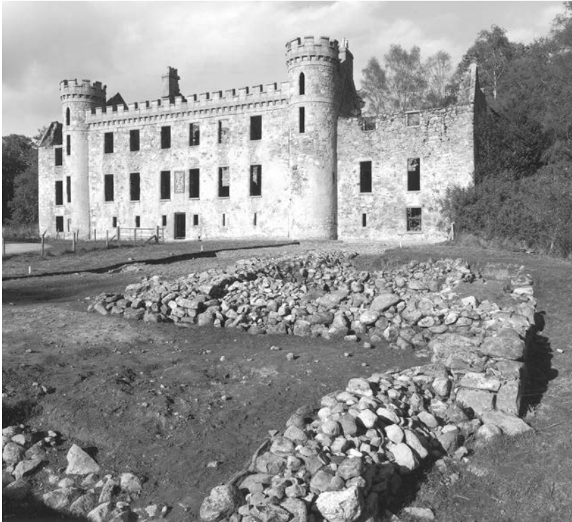
ILLUS 1 Fetternear House, Aberdeenshire, in 1995, with the excavated remains of the bishop's palace in the foreground ( Crown copyright: RCAHMS )
