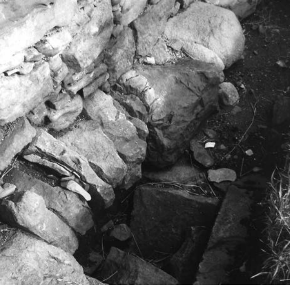
ILLUS 9 Garderobe outfall at the foot of the south wall
