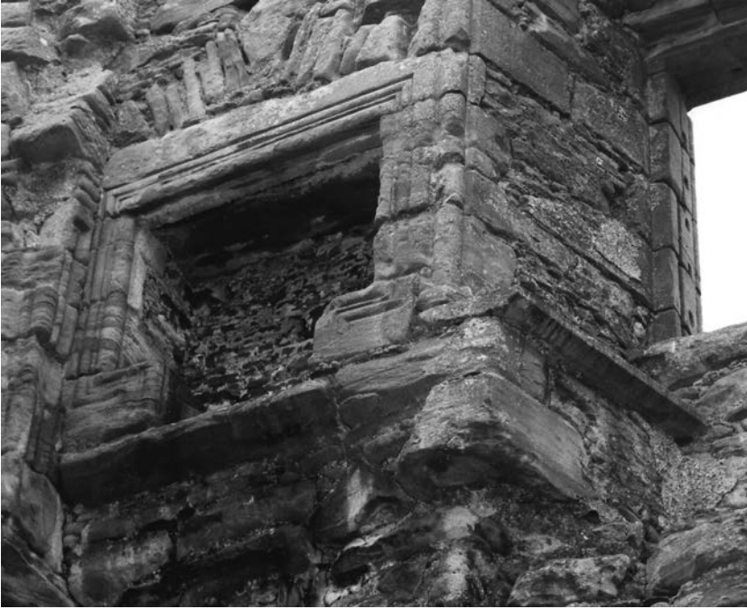
ILLUS 6 Aumbry in the south-east corner of the second floor beside a window with the sliding shutter feature, the broad groove for which can be seen
