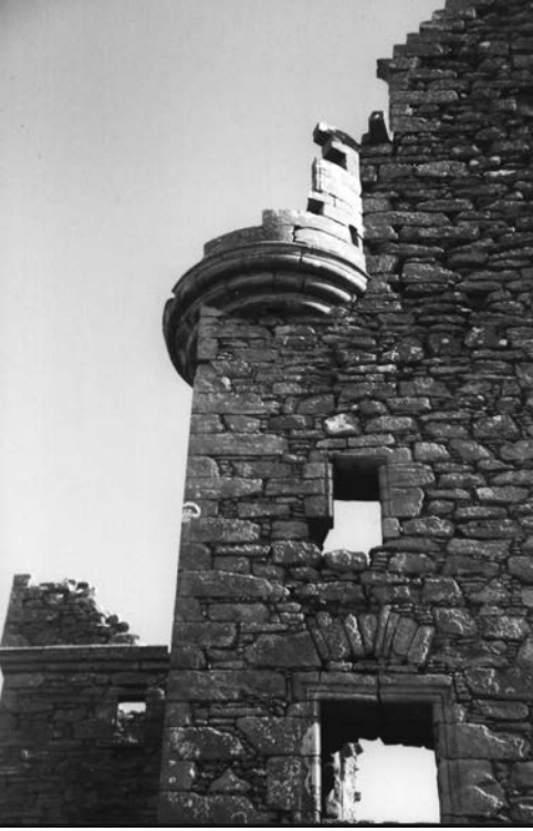
ILLUS 7 Turret at the north-west angle viewed from the west
