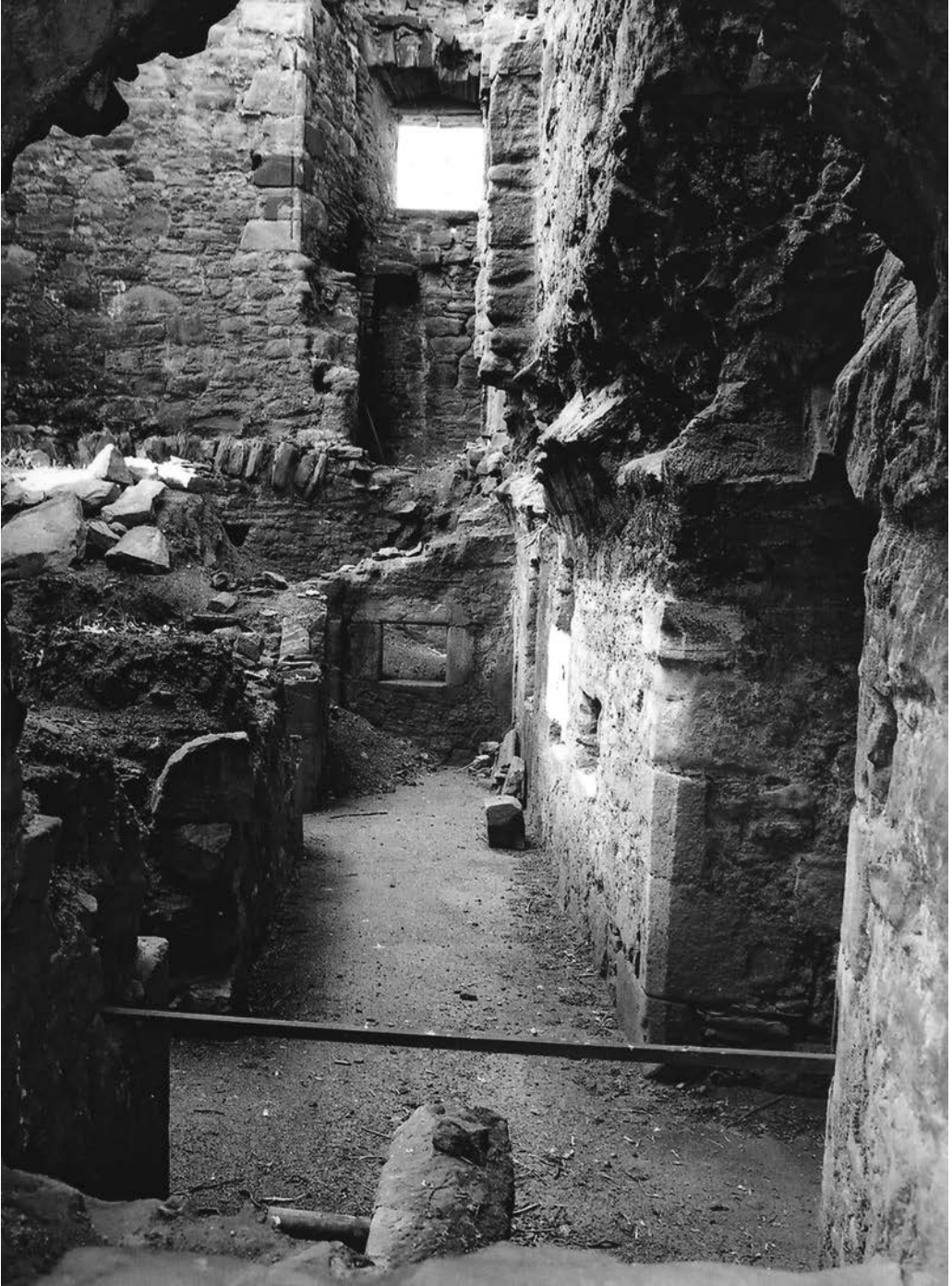
ILLUS 3 View of corridor looking west, showing serving hatch to the kitchen. The wooden bar has been inserted in the window embrasure dook holes to illustrate an apparent device for restricting access
