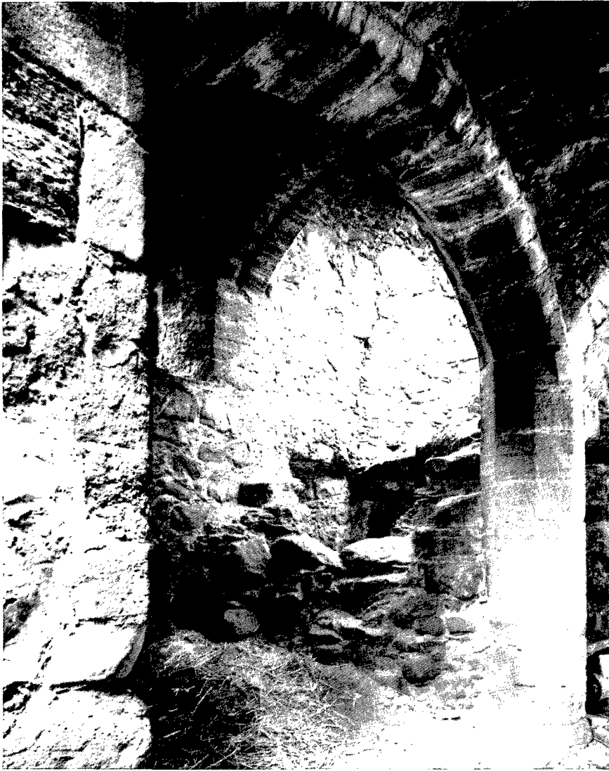
ILLUS 2 The interior of the great stair. The magnificent dressed stone would have been offset against plaster, thus highlighting the sunk carvings.
