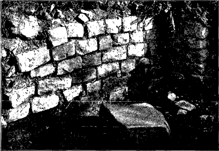
Fig. 21. South-east Corner, interior of Butressed Building, showing Doorway built up.
