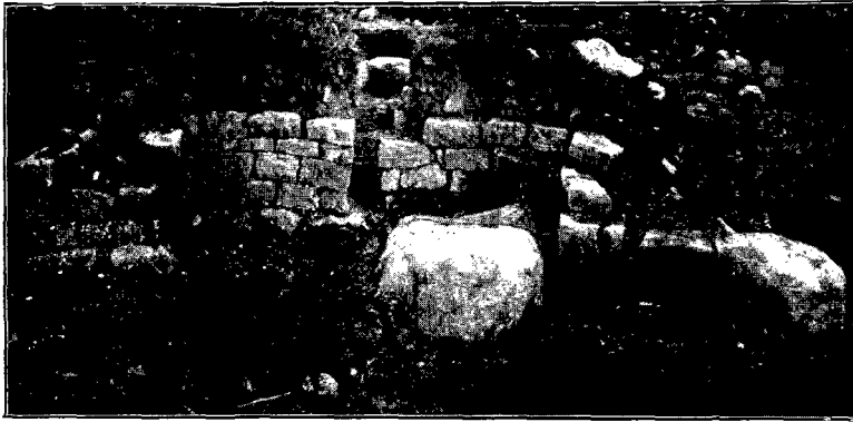
Fig. 18. Outer Face of the East Wall of Buttressed Building, showing buttress built between two large boulders.
