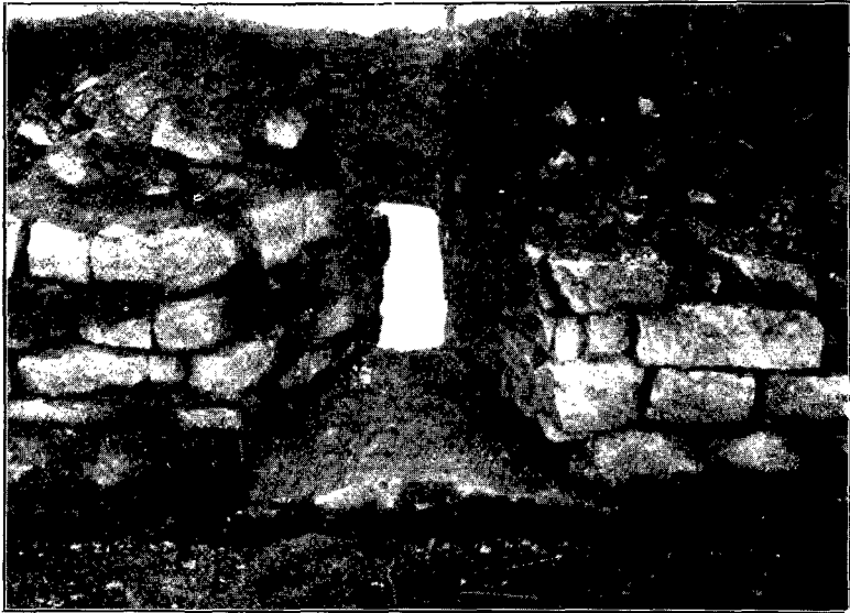
Fig. 20. Interior of Buttressed Building, showing opening in wall. East side.
