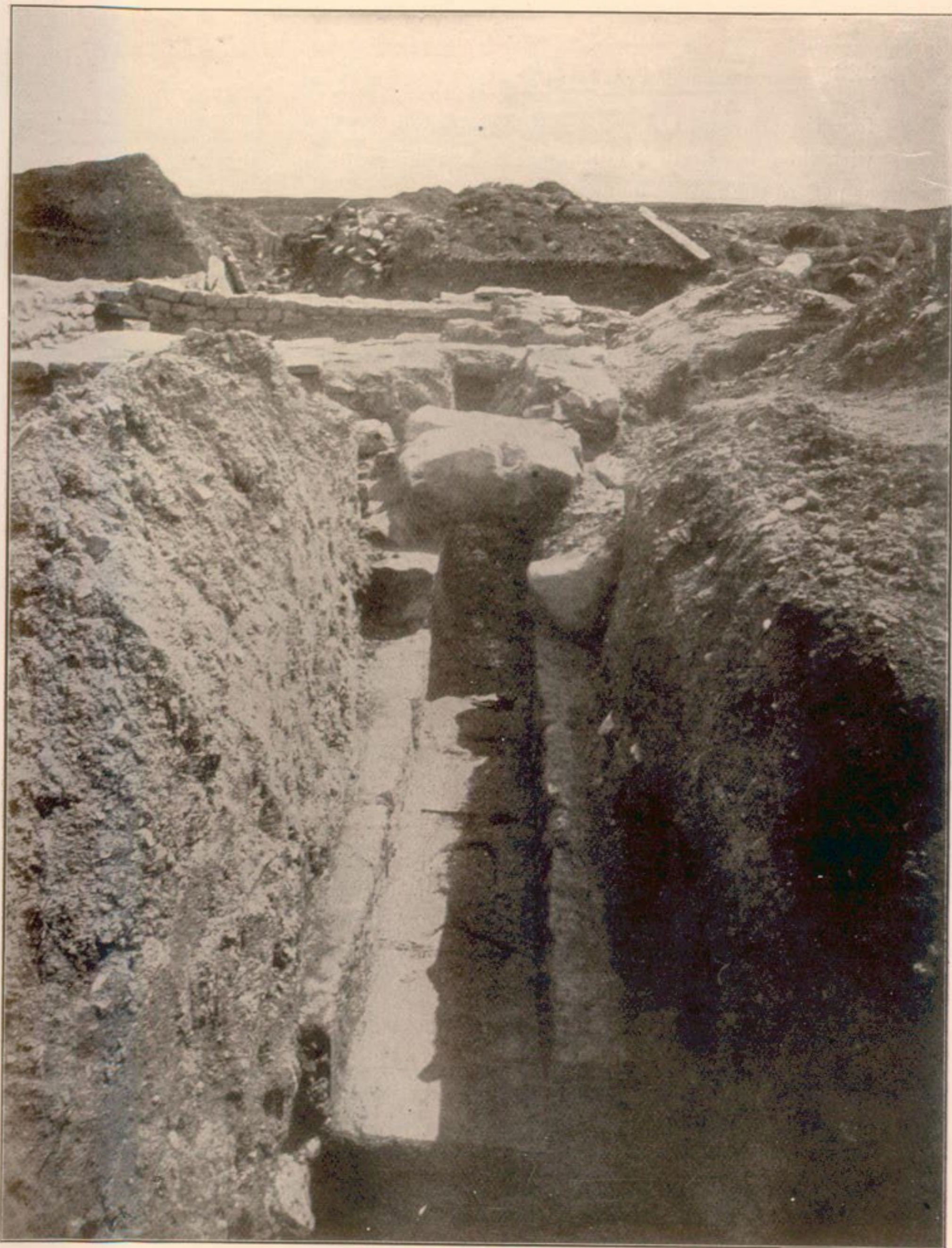
Fig. 26. Conduit through north wall.
