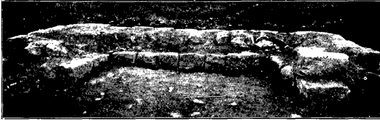
Fig. 24. South-west Corner Tower.
