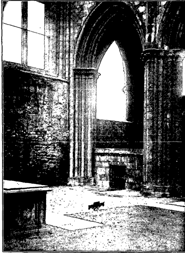
Fig. 1. View of entrance to the Stuart Tomb, showing also the gravel walk in front, where the second-found remains from Trinity College Church were re-interred. (From a photograph by C. W. Sinclair.)
