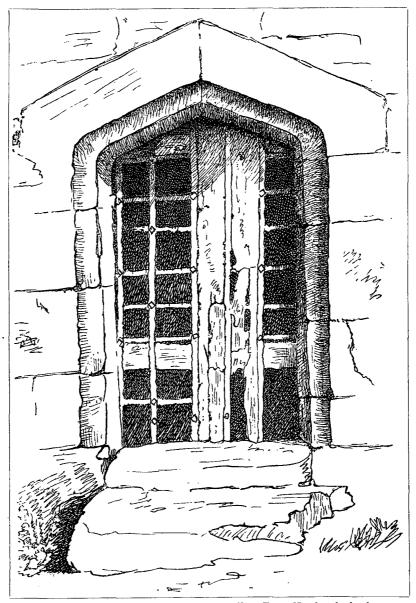
Fig. 23. Grated and Planked Door, Bywell-on-Tyne, Northumberland.
